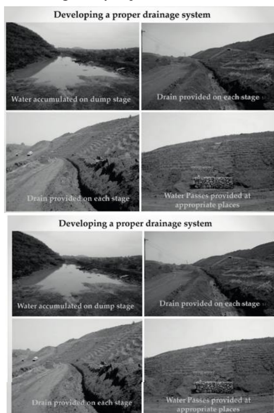
Pic-4: Drainage system on Mine dumps
